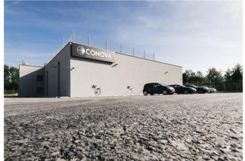
Salzburg South: Data Center 6 & 7 in Hallein
